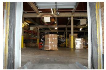
RF Controls' smart antenna (circled in red) tracks product as it is loaded onto a truck, eliminating the need for manual scanning to record supply chain activity.
